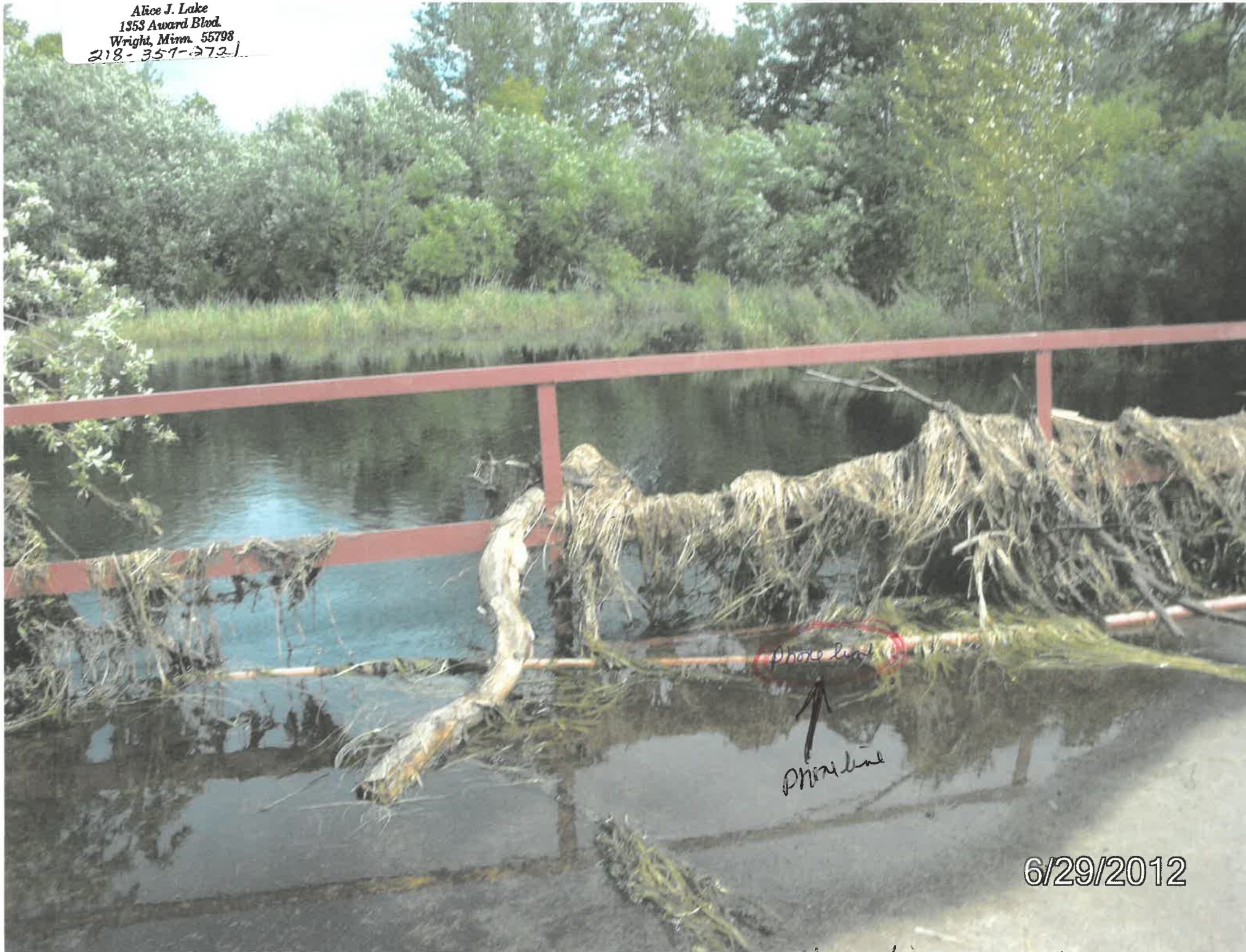
Recent flood Carlton County Phone line Across Tamarack River
